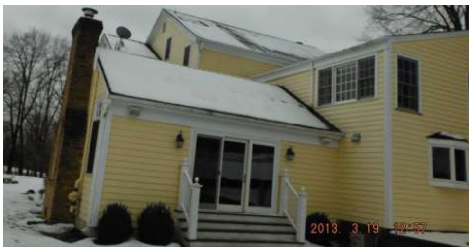
Figure 6 Snow cover; partial view during the day as snow changed to freezing rain. Recommend more ventilation on all roofs; poor or inadequate.
