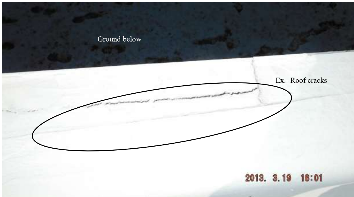
Figure 28 Example of cracks on roof; leaking and poor condition/very old and patched.
