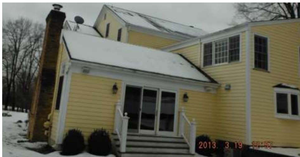
Figure 32 Snow cover; partial view during the day as snow changed to freezing rain. Recommend more ventilation on all roofs; poor or inadequate.
